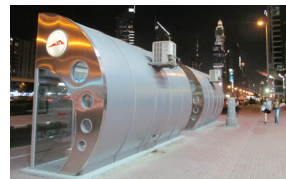
Bus Stop with A/C in Dubai, UAE
