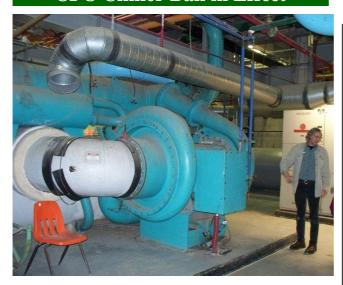
Both the Province of Manitoba and Government of Canada have current bans on the use of chillers using any CFC, such as R-11 or R-502. All CFC refrigerant containing chillers must be permanently shut off (i.e. decommissioned or retrofitted) never to run again with a CFC. December 31, 2014 was the deadline set in stone in the Manitoba Ozone Depleting Substances and Other Halocarbons Regulation 103/94, as well as, under Canada's Federal Halocarbon Regulation.
